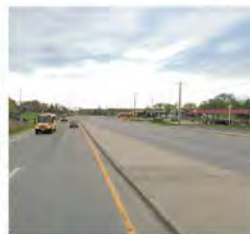
Tom Watson Parkway (Expressway) looking east at 9 Highway
