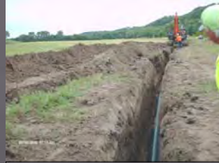
Open trench across PLP..
