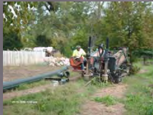
Drill rig, bored under Main St.
