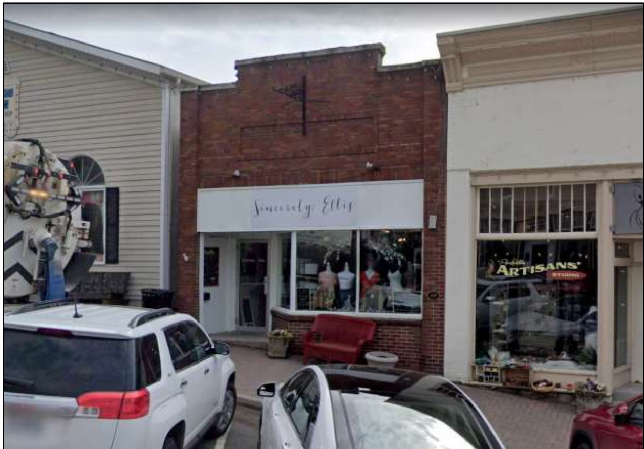
Imagery of 113 Main St. (dated May 2019, prior to exterior improvements)
