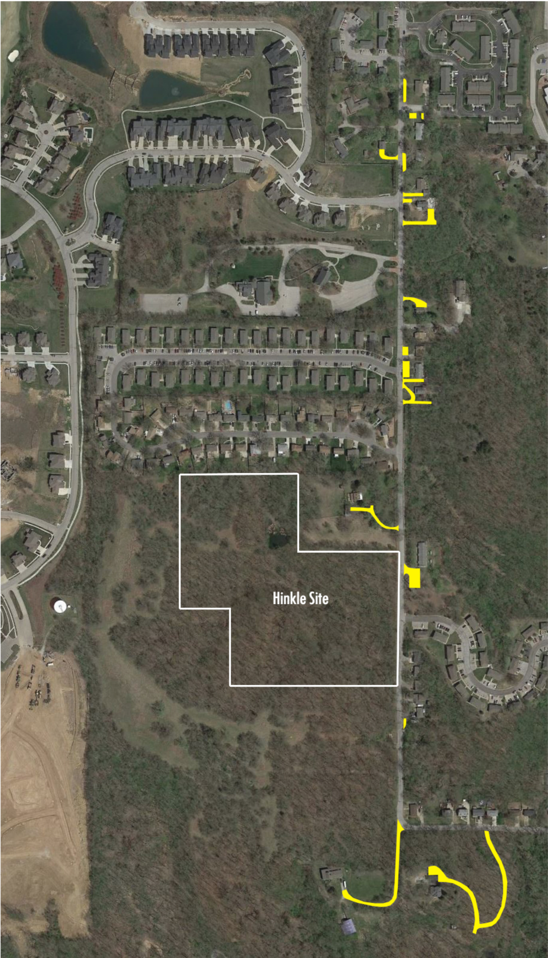
(15) Gravel Driveways Along Bell Road, Currently
