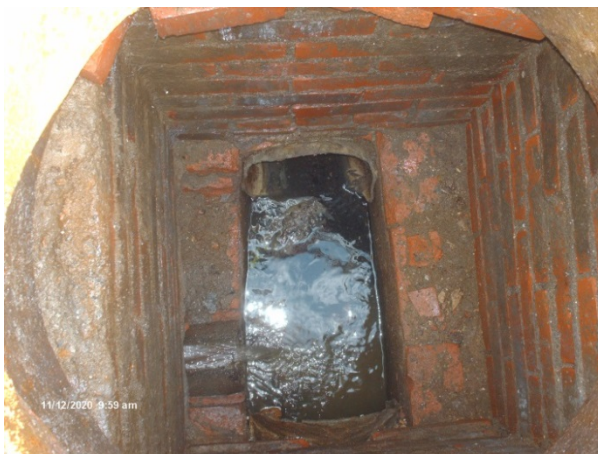
Typical brick "box" MH, in Hwy 9.
