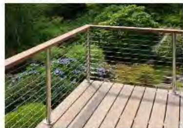
Decking & Aluminum Railing
