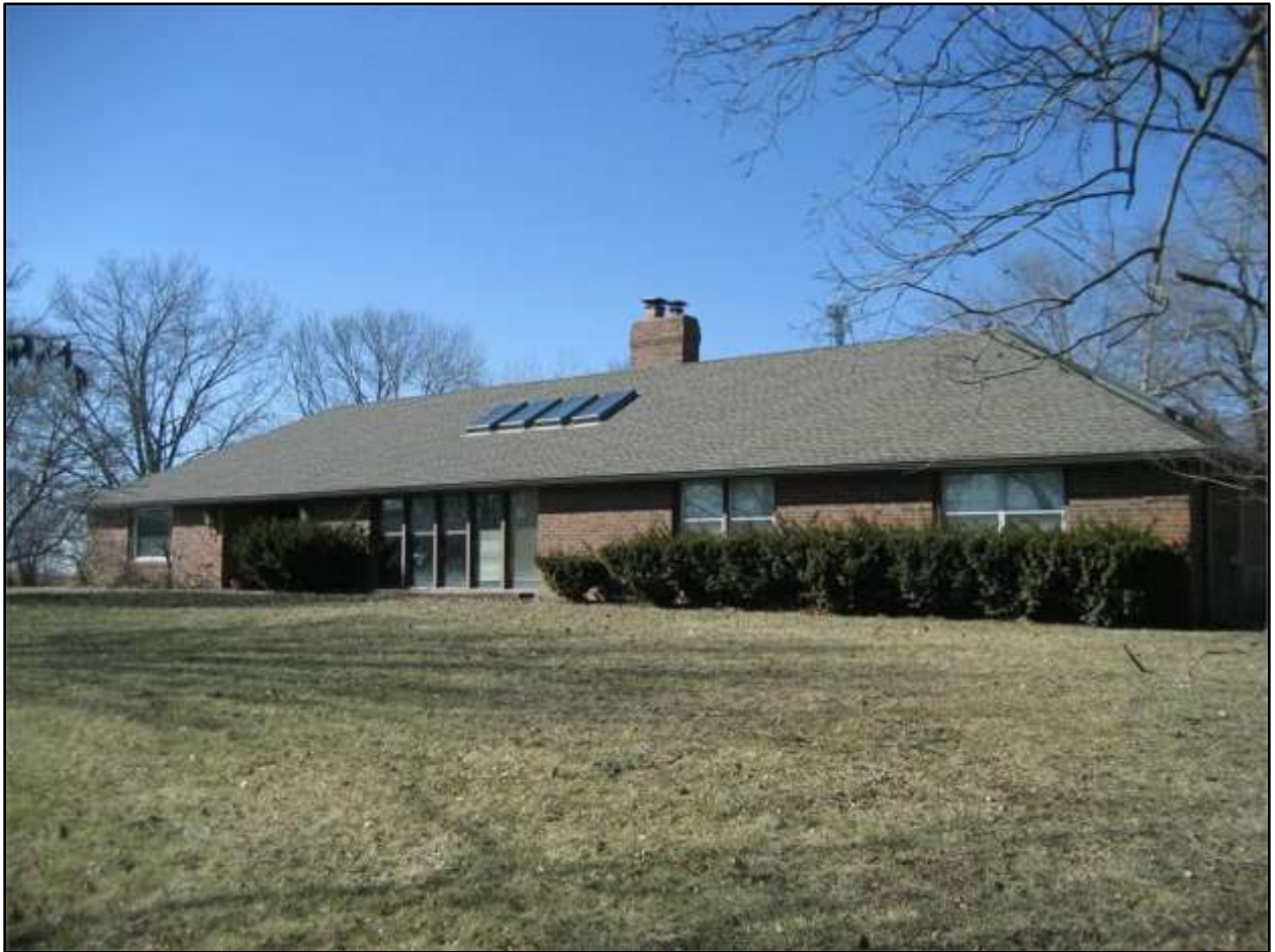
Photo courtesy of the Platte County Assessor's Office
