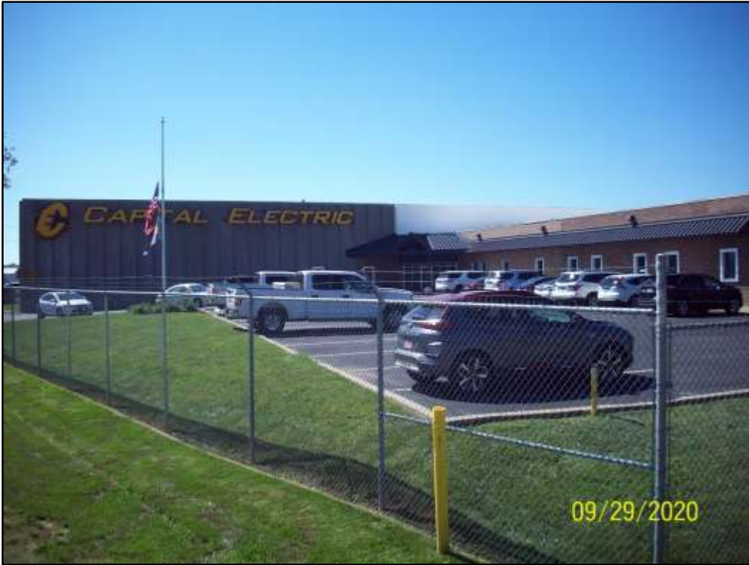
View of Capital Electric building looking towards the southwest
