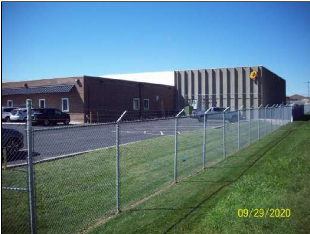
View of Capital Electric parking lot looking towards the west
