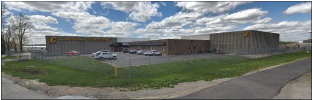
Panoramic view of Capital Electric Building looking towards the southwest
