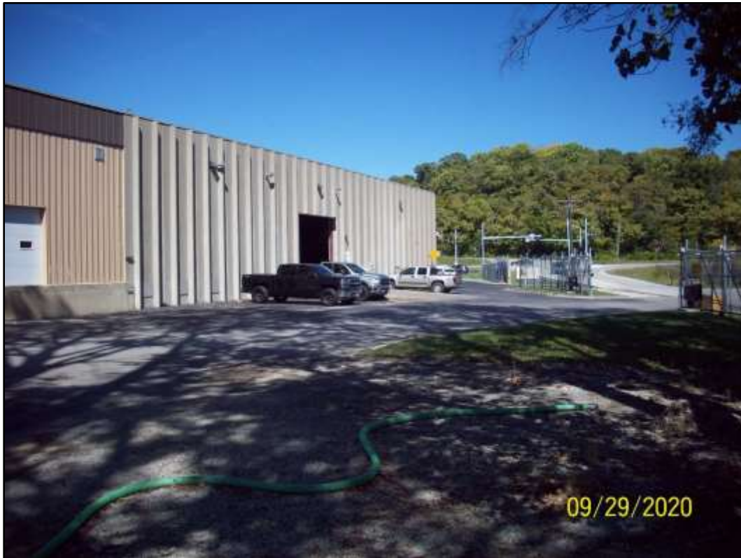
View of Capital Electric warehouse looking towards the north
