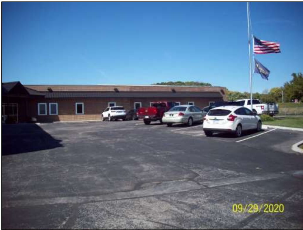
View of Capital Electric parking lot looking towards the west
