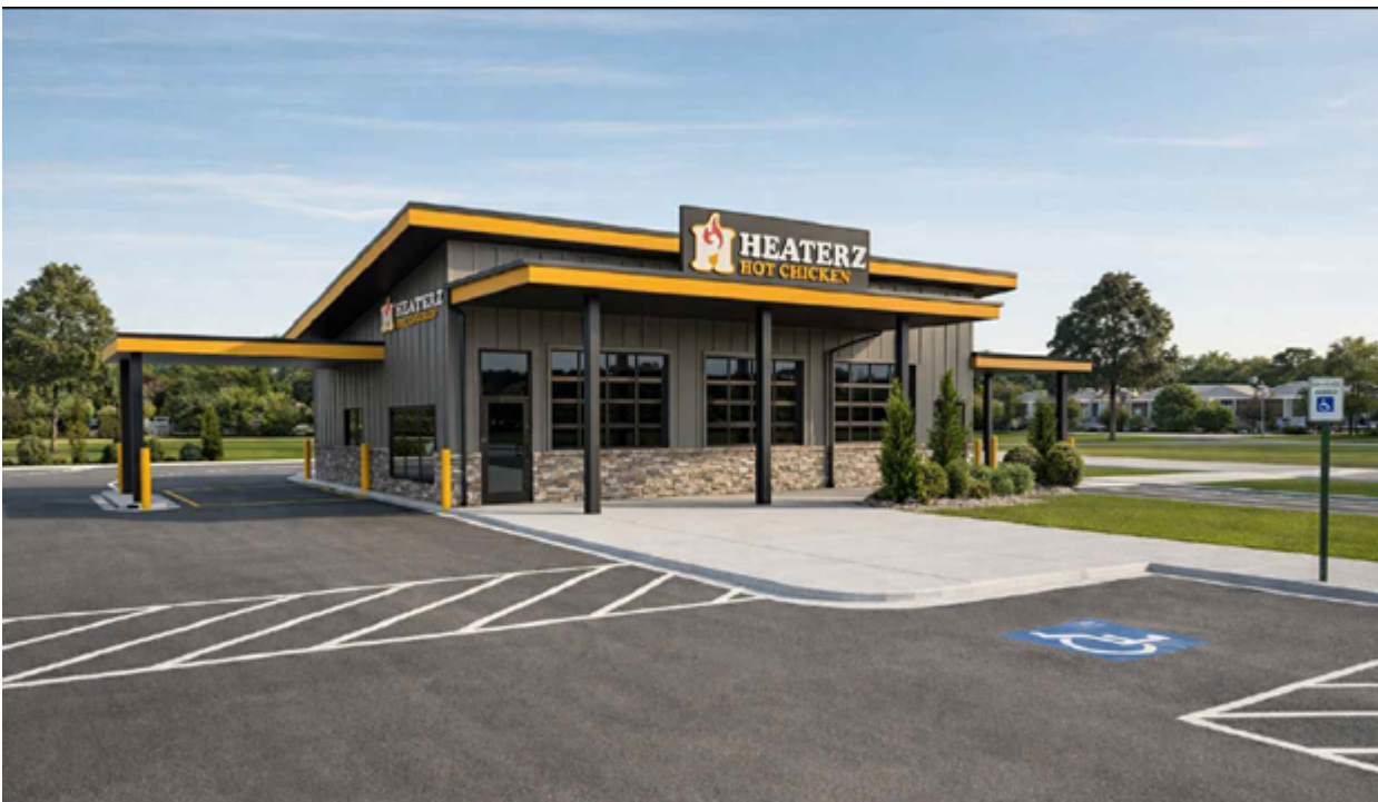
View of Heaterz eastern elevation façade
