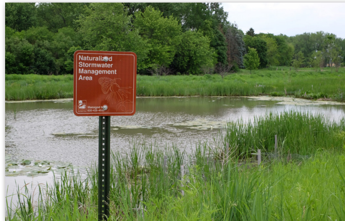
Naturalized detention basin
