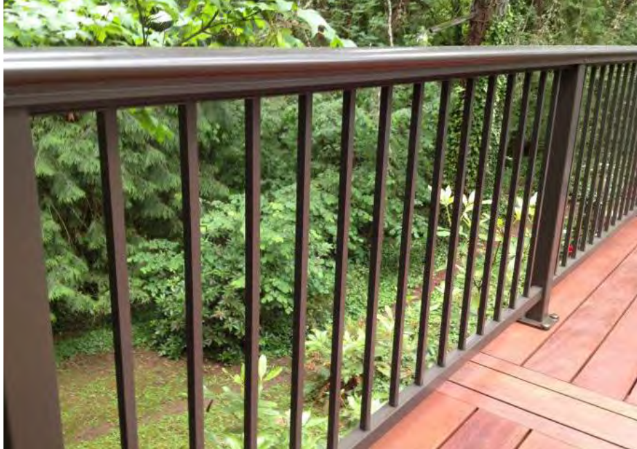
Decking & Aluminum Railing
