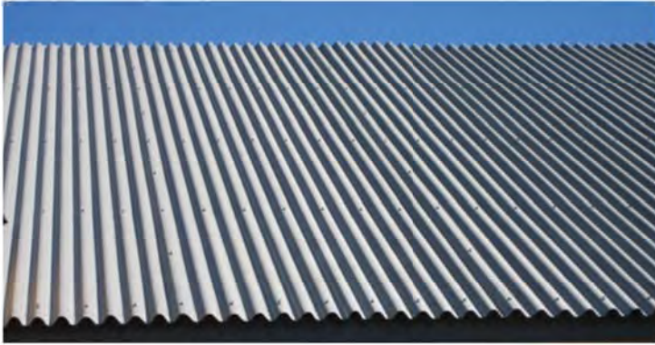
Corrugated Metal Roof
