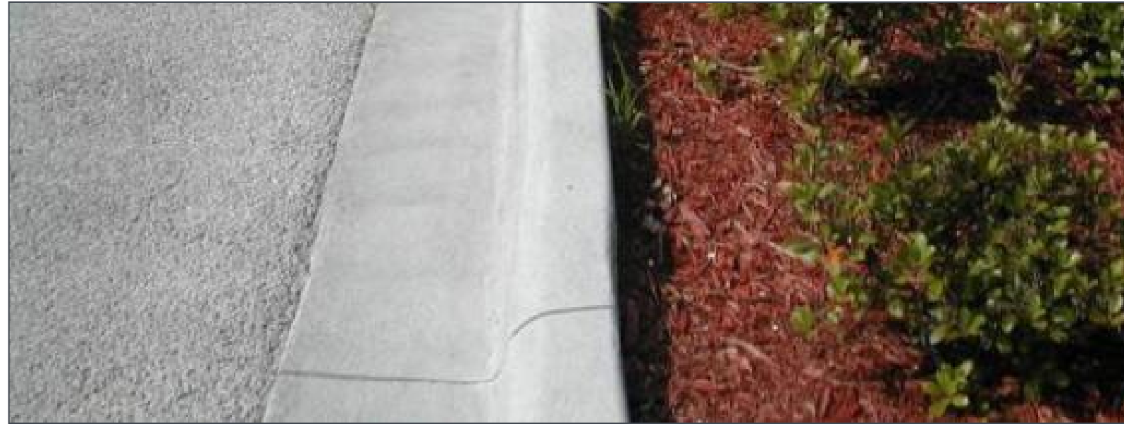
Barrier curb with grade separation
