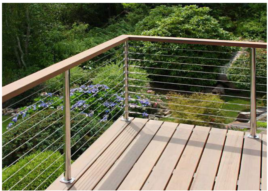
Decking & Cable Railing
