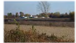
Parkville Sewer Plant
