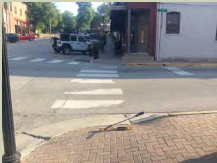
Curb Ramp Cross Slope
