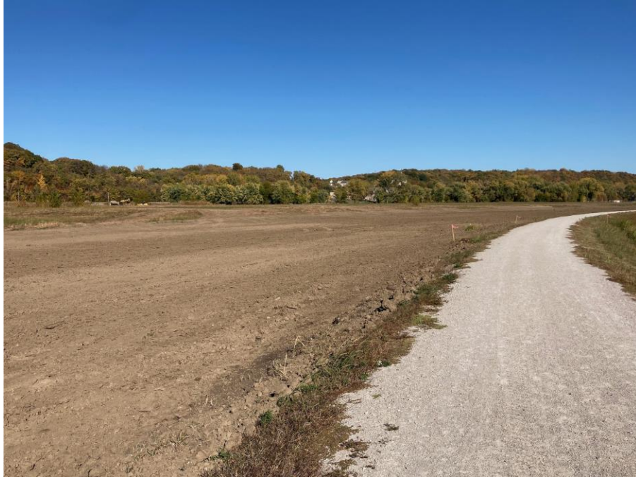
October 21, 2023. Clay has been spread across the bottom of the wetland. North basin, looking northeast.
