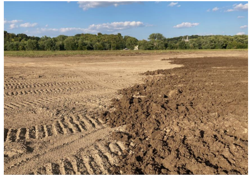
September, 2023. Placing clay over the wetland basins. Underlying soil is on the left, clay on the right. North basin, looking northeast.
