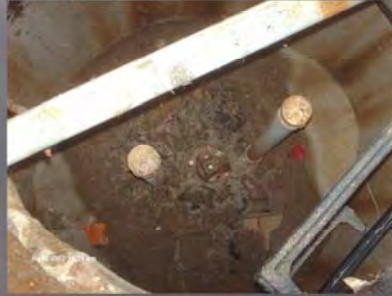
Utility bore through pit.
