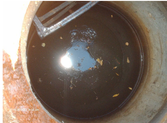
Some pits fill with groundwater. Hard to prevent. Makes access more difficult.
