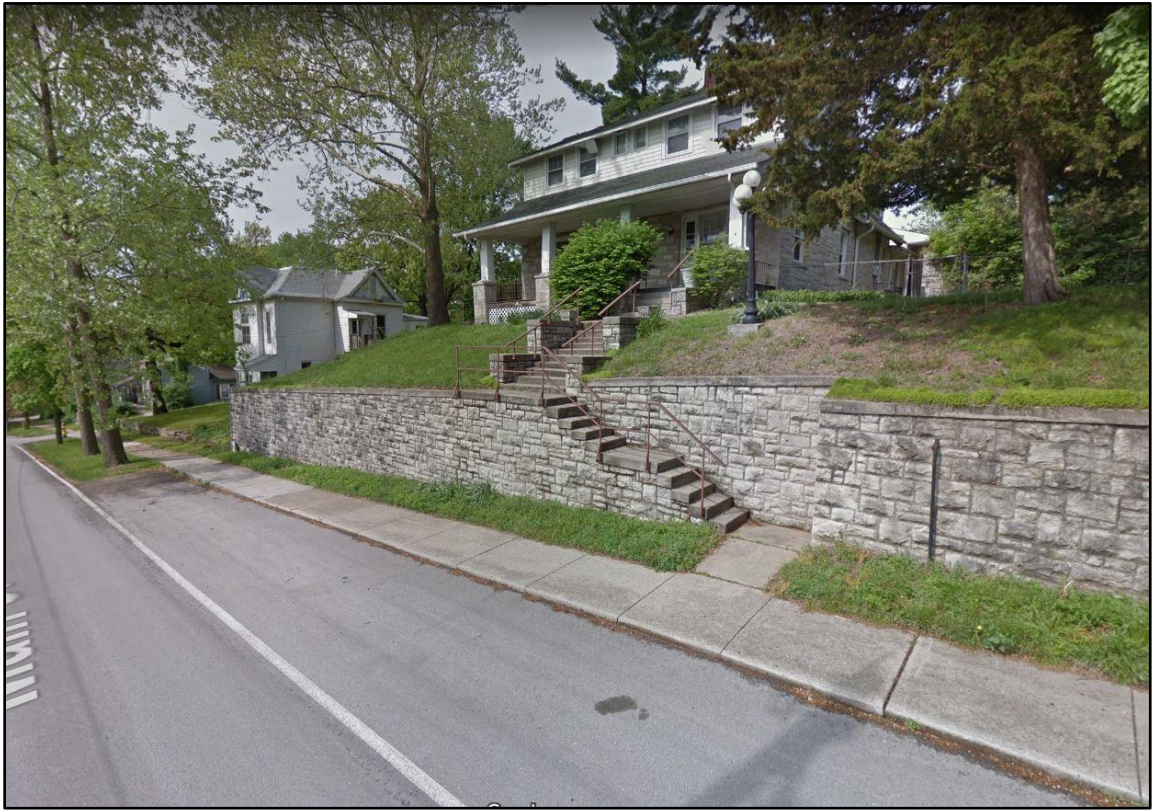
View of on-street public parking along 804 Main St.
