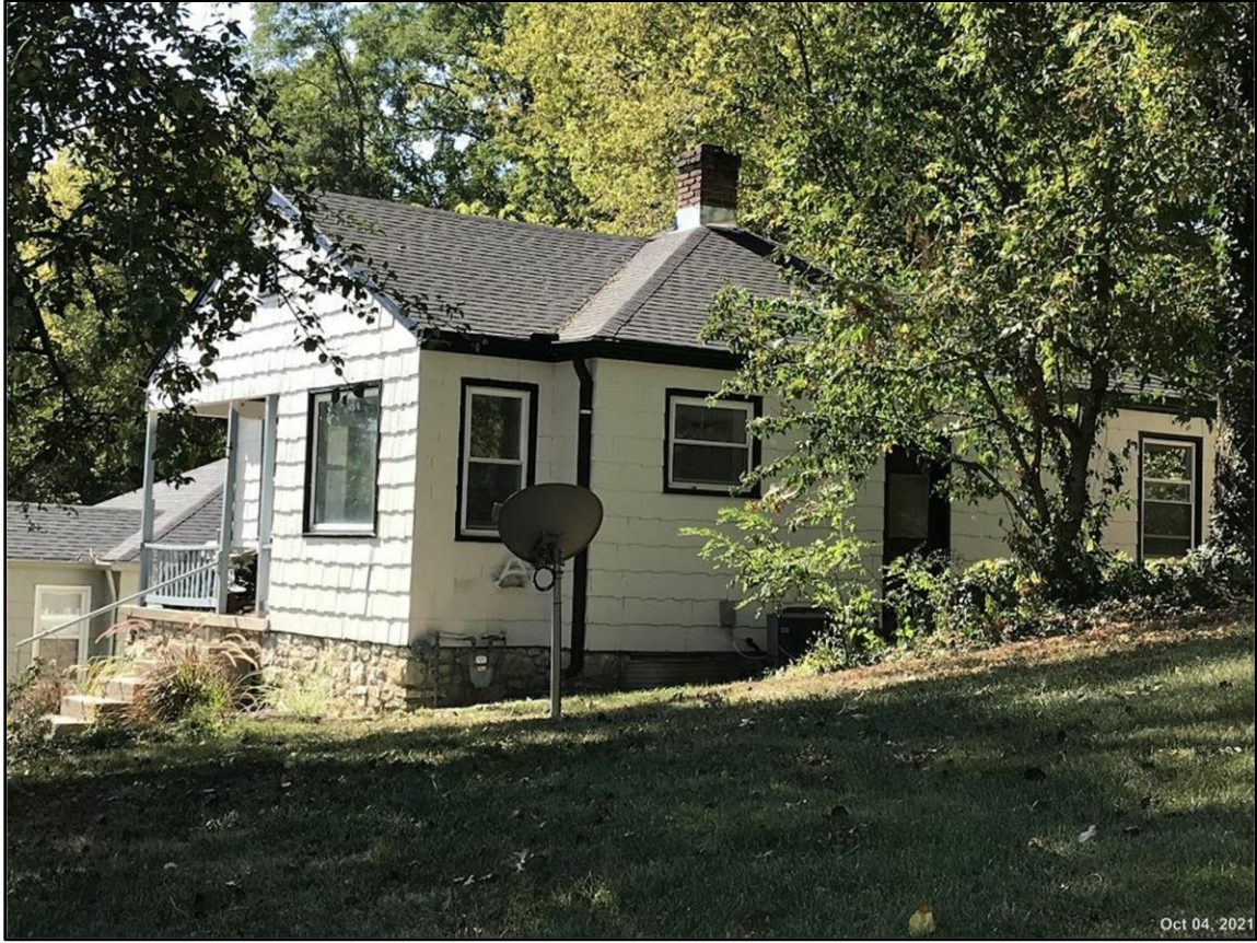
View of 826 East St. (looking towards southwest) from W 12 th St.
