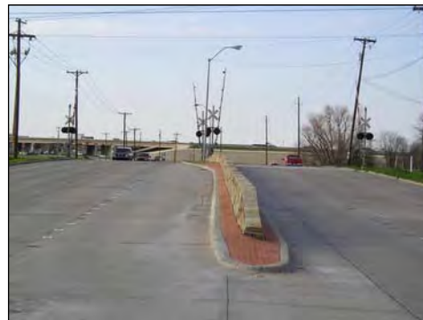
Roadway Channelization and Median Barriers
