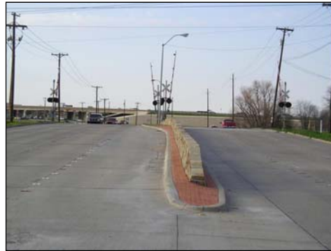
Roadway Channelization and Median Barriers
