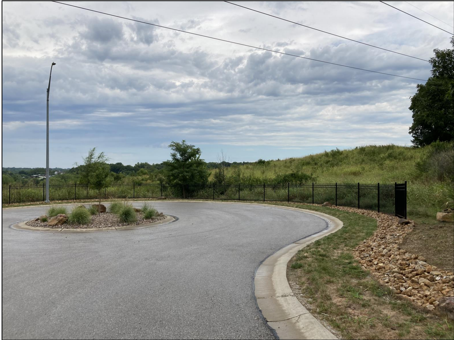
View of Lime Stone Ct traffic circle looking towards the northwest
