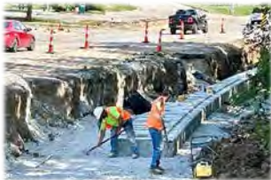
Crews install retaining wall
