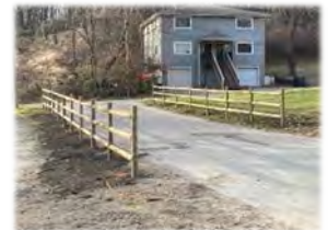
Fence installed at entrance
