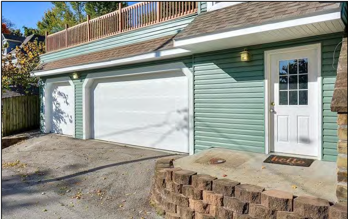
View of garage parking along 11 W 5 th St. private alleyway.
