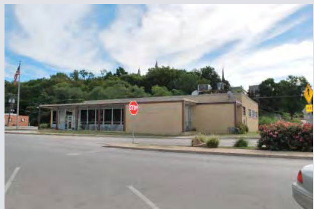
Fig. 3.56 & 3.57 – Views along East Street/9 Highway.
