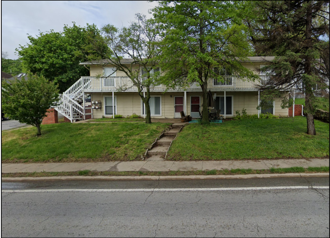
View of 500 East St. (looking towards the west) from Missouri Hwy 9
