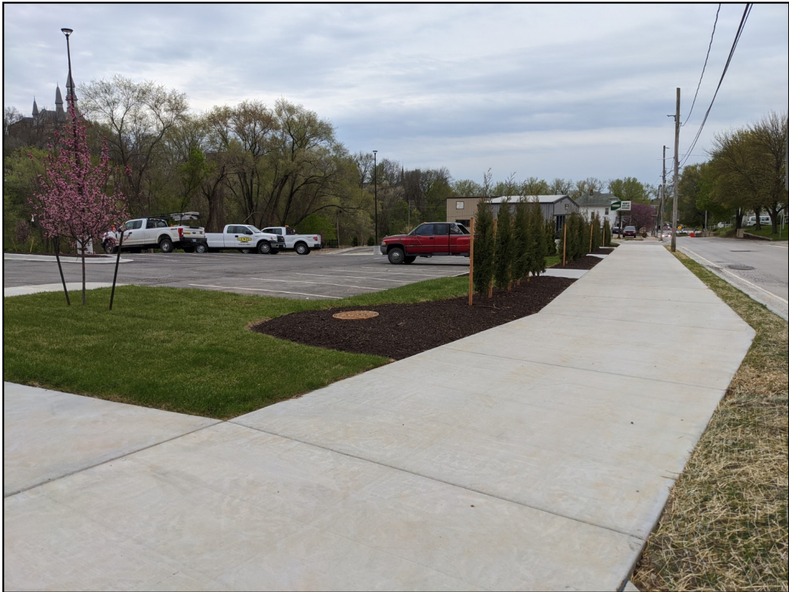
View towards public parking lot spaces at 603 East St.
