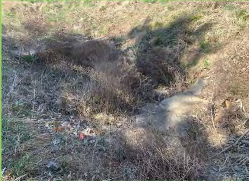
Inside of Culvert up close of brush to be cleared
