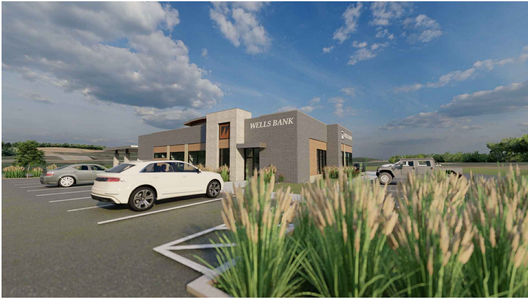
View From Southeast Corner
