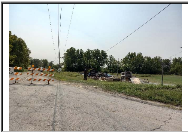
View to the east towards the closed Brush Creek Bridge
