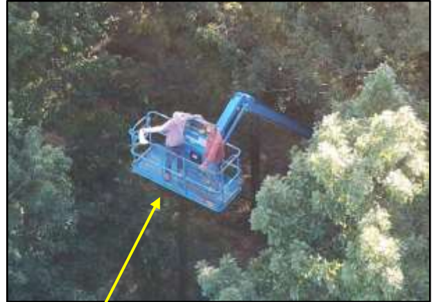
Don Julian in power lift bucket (height approximately 65 ft.)
