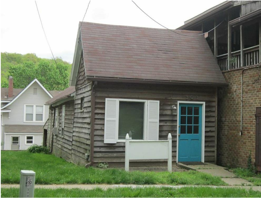
Photo courtesy of the Platte County Assessor's Office
